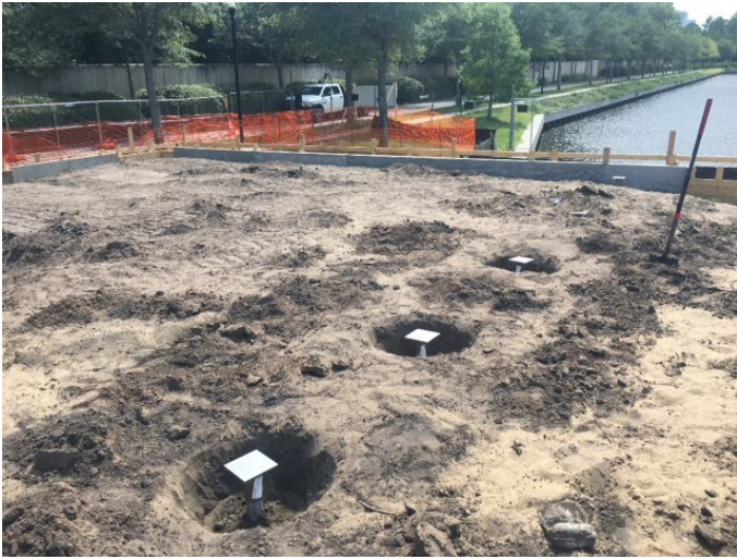
Pile caps installed to allow for pile and footing connection.
