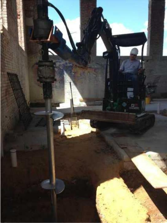
Galvanized 10,12,14 lead section being advanced by MGF owner, Mason Frascona. Digital Torque Indicator mounted between the drive head and drive tool.
