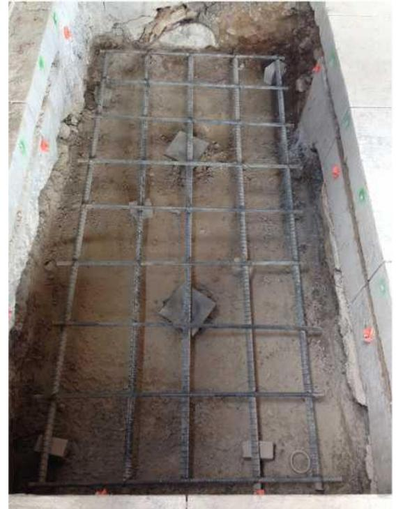
7x7x0.5 new construction pile caps set at elevations 3 inches from bottom of footing.
