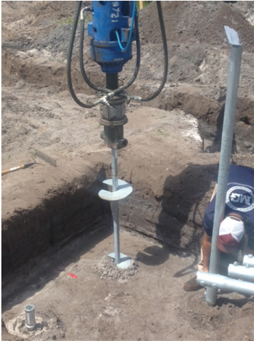
Square shaft lead section installation (back left) Round shaft extension bolted to lead section (right) Square shaft to round shaft transition fitting (front left)
