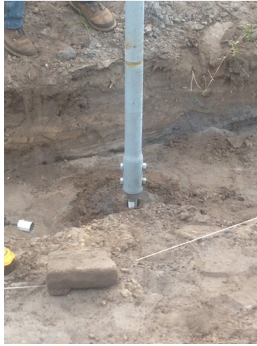
Square shaft to round connection
