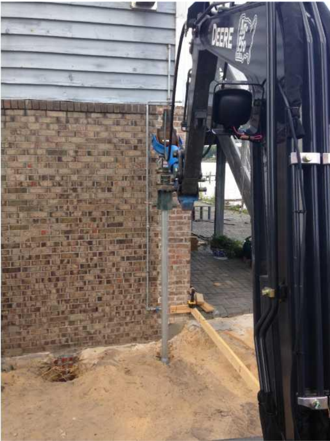
Helical Pile advanced adjacent to existing foundation.
