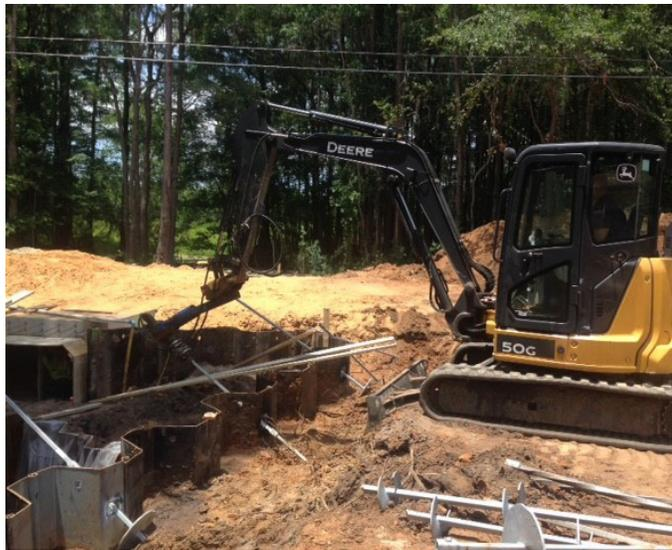
Anchor Installation through Steel Sheet
