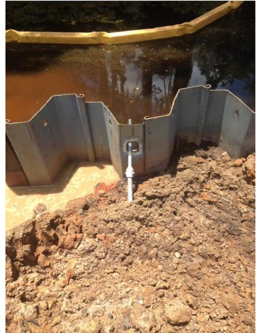
Anchor with Thread Rod Adapter to allow for sheet connection
