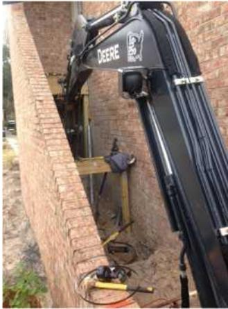
Underpinning pile installed below landing
