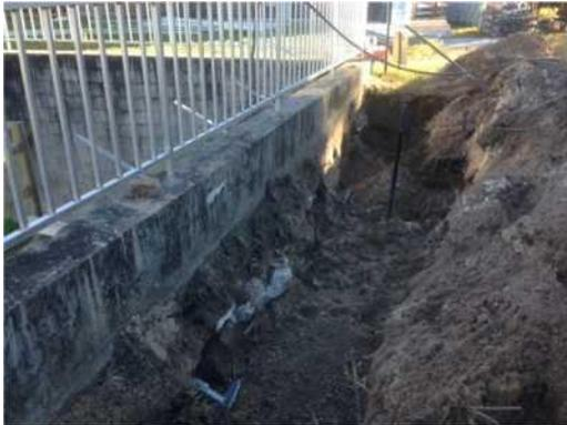
Soil excavated behind wall to allow anchor leads to be installed behind wall. This prevented the need for larger holes cored in the block wall.
