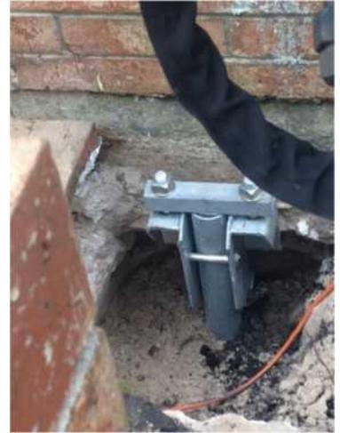
Retrofit bracket attached to existing footing
