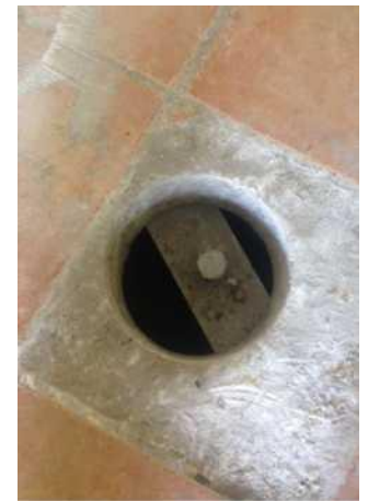
Top view of slab lifting bracket
