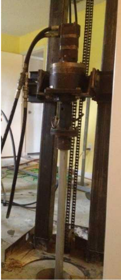
Mobile drive head installing pile
