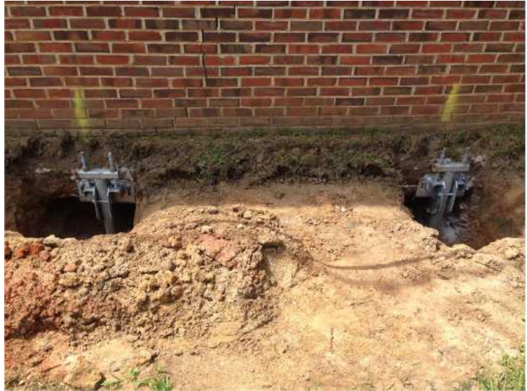
Completed underpinning system
