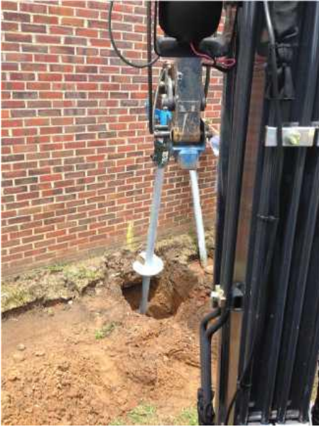
Advancing helical lead section
