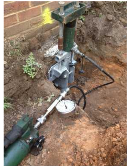
Setting each bracket to the design load
