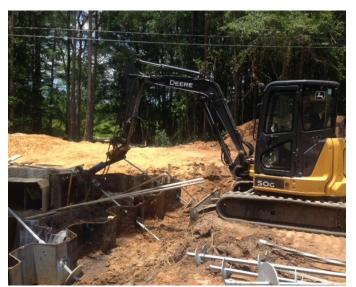
Anchor Installation through Steel Sheet
