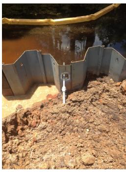
Anchor with Thread Rod Adapter to allow for sheet connection
