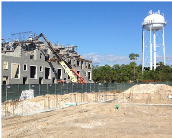
View of the work site in relation to structure under construction.
