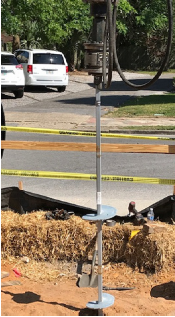
Installing the pile
