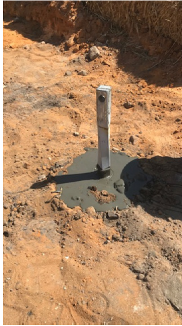
Grout encased pile shaft
