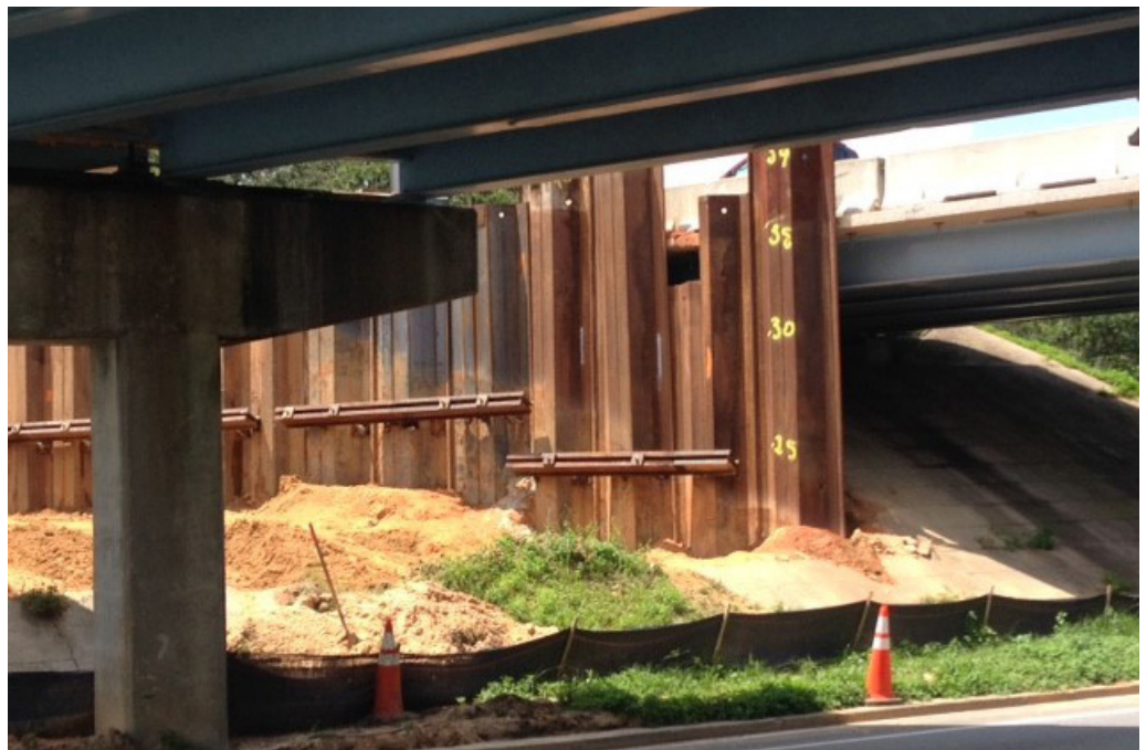
View of the work area and existing roadways.
