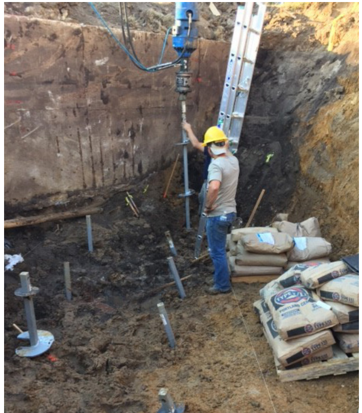
Installation of the helical lead section
