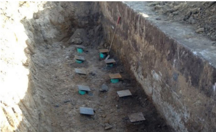
View of completed pile system
