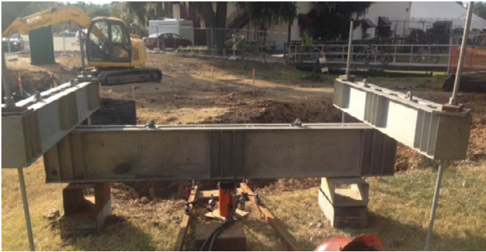
Vertical Load Test
