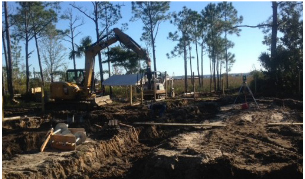
View of the work area and installation equipment
